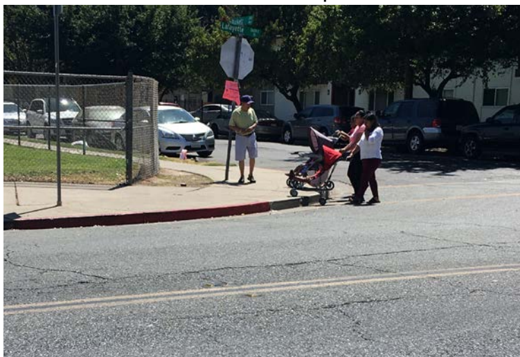
Parent navigating lack of curb ramp with stroller.
