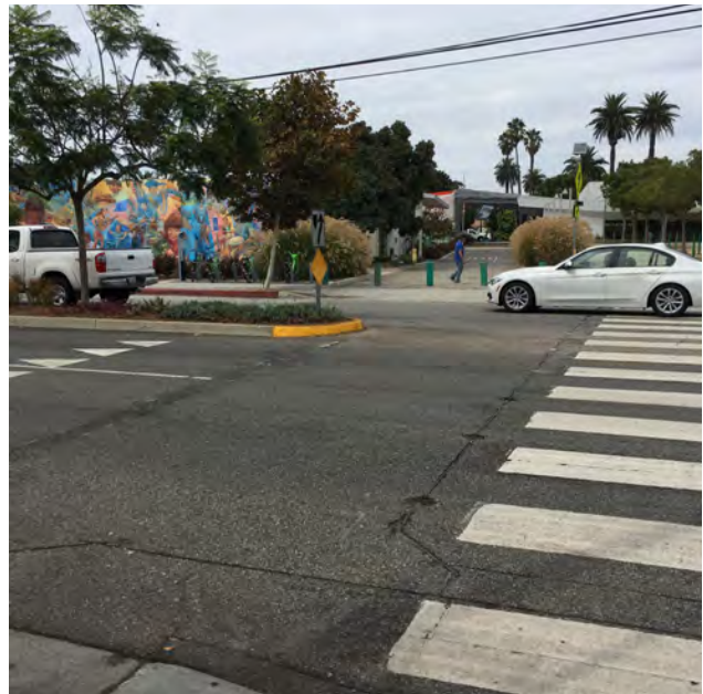
Left: The color has faded from the crosswalks at the Pico Boulevard/20th Street intersection.
