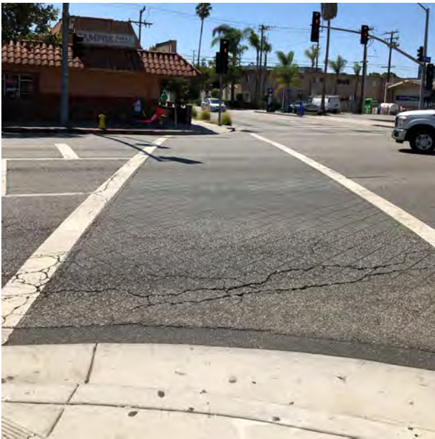
Left: The color has faded from the crosswalks at the Pico Boulevard/20th Street intersection.
