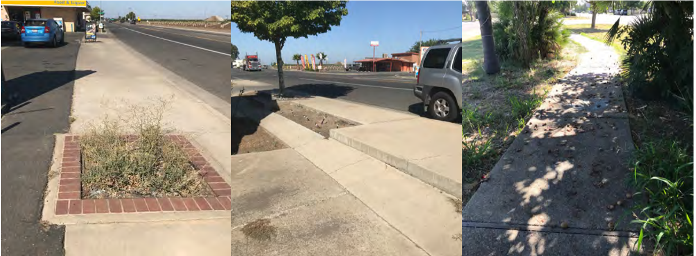
Left: Various large and unmaintained tree wells along Central Yosemite Highway take up the majority of the sidewalk space. Center: An uneven sidewalk leading to San Joaquin Drug Store on the southside of Central Yosemite Highway and Sutter Street presents a tripping hazard to pedestrians. Right: Debris on pedestrian pathway on Broadway.
