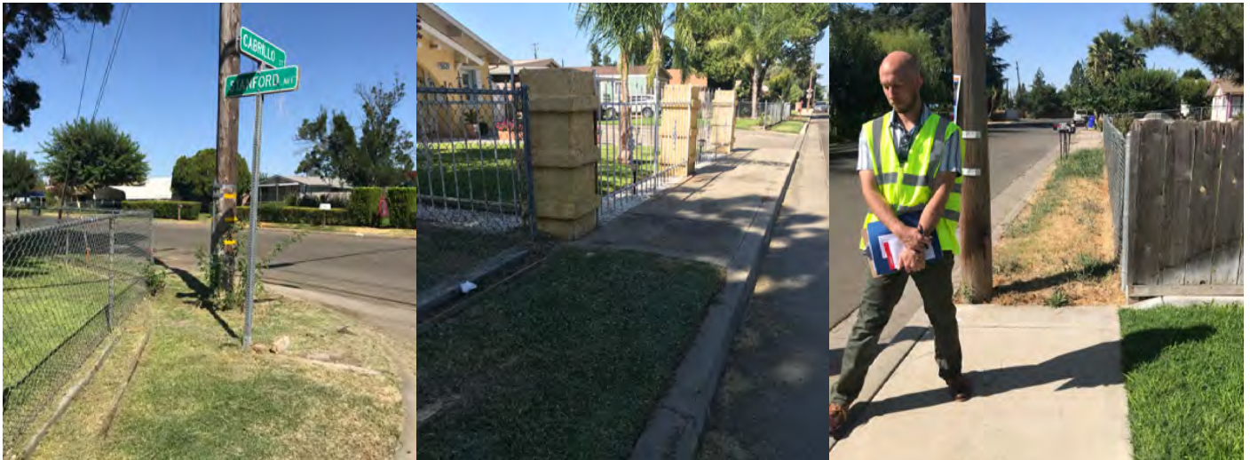
Left: No sidewalk or curb ramps on the corner of Cabrillo Street and Stanford Avenue. Center: Discontinuous sidewalks along Stanford Avenue. Right: Patchwork sidewalk network on Carson Street creates navigation challenges for all.
