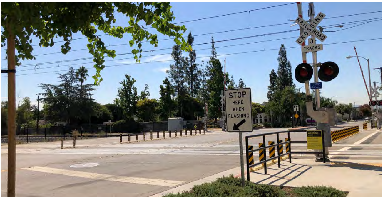
Railroad crossing gates impede motorists but not pedestrian traffic on the sidewalk when a train is approaching.
