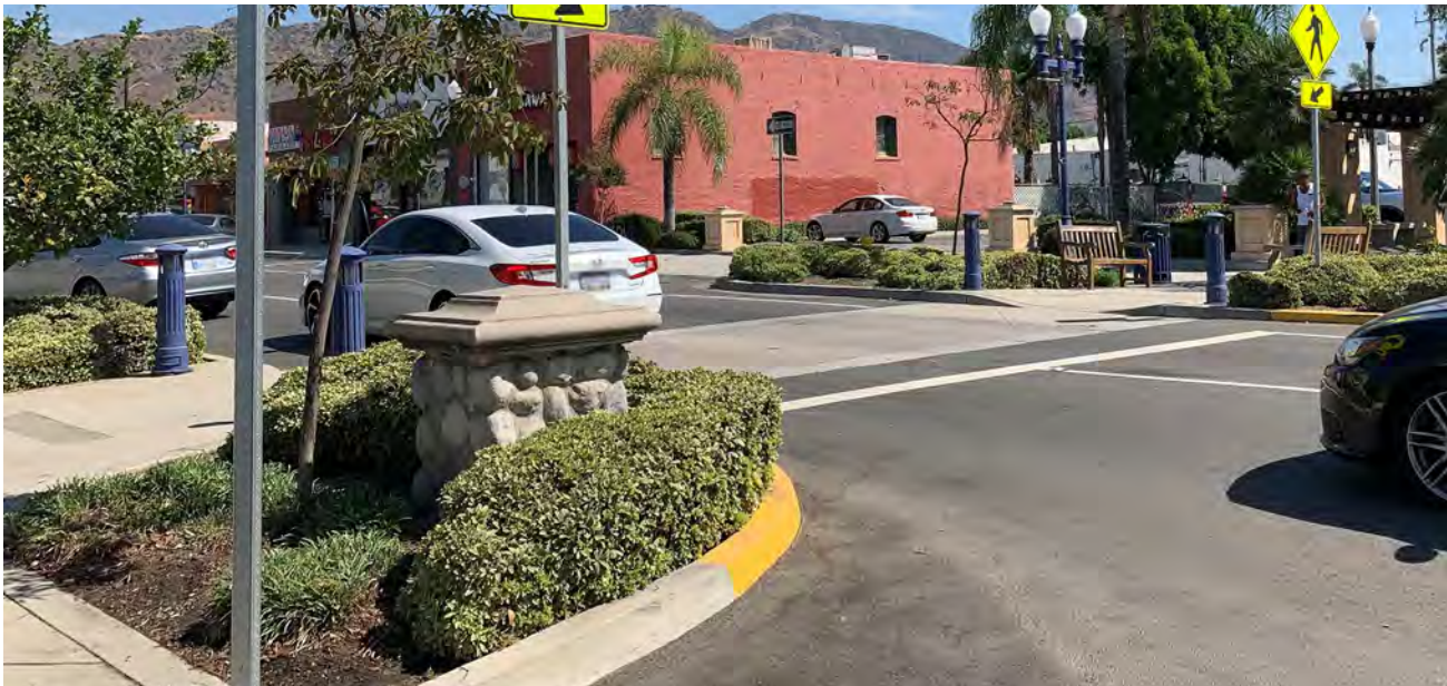
Top Left: West Foothill Boulevard and East 5th Street crosswalks lacks stop lines stop bars; this adds to unsafe conditions for all road users. Top Right: Various road users travel across North Azusa Avenue and West Foothill Boulevard where there are no stop bars that clearly demonstrate where cars should stop. Bottom: Bulb outs along North Azusa Avenue between West Foothill Boulevard and East Santa Fe Avenue adjacent to the CVS shorten the crossing distance for pedestrians.
