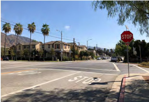
Left: Standard crosswalk markings at the Alameda Avenue/East 9th Street intersection. Right: This crosswalk leads to the Metro Transit Center and is on the east side of the North Azusa Avenue intersection and lacks stop bars. Stop bars indicate to drivers when they should stop to allow pedestrians enough space to cross.
