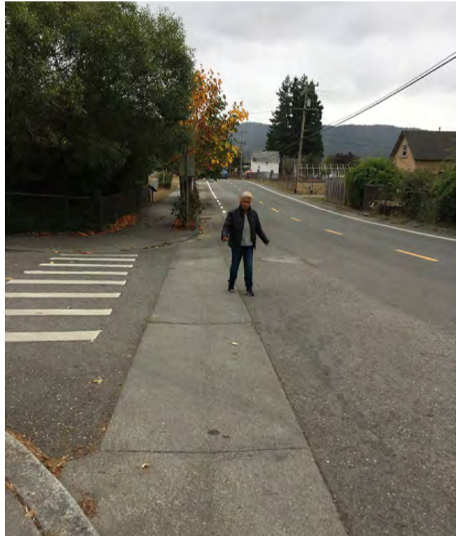
Left: Missing curb ramps at the intersection of Broderick Lane and South Railroad Boulevard.
