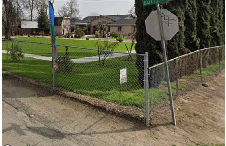
Dirt paths instead of sidewalks at the Sutter Avenue/Elsie Street Intersection.
