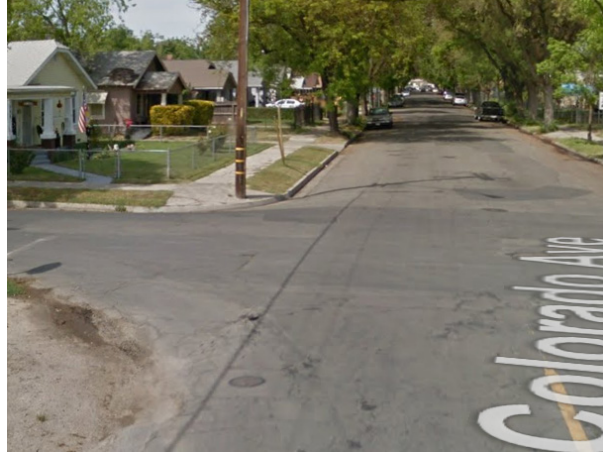
Pedestrians often wait a long time for drivers to yield at the Colorado Avenue leg of the Colorado Avenue/South Avenue intersection.
