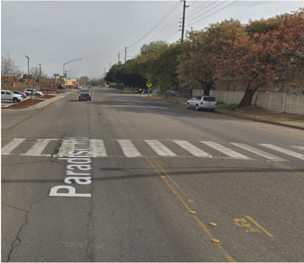
The ladder crosswalk markings along Paradise Avenue, at Florette Avenue (left) and Sheridan Street (right) are faded.
