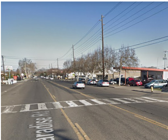
The northern crosswalk at the Paradise Avenue/Chicago Avenue intersection leads pedestrians into parked cars on the west side and drops them off into the street on the east side.
