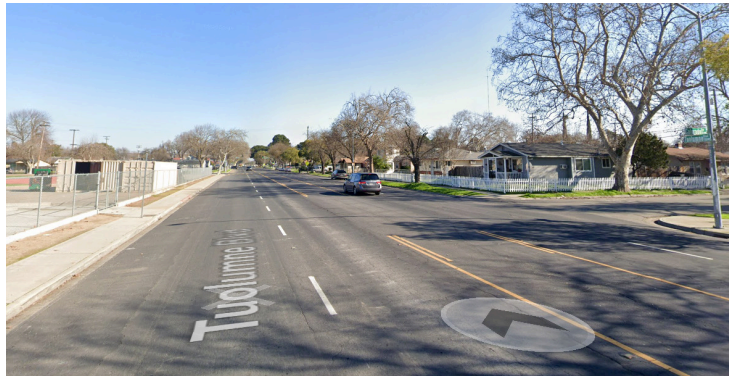
There is no signage or indicators to drivers that pedestrians might be crossing at the Colorado Avenue/Tuolumne Boulevard intersection.
