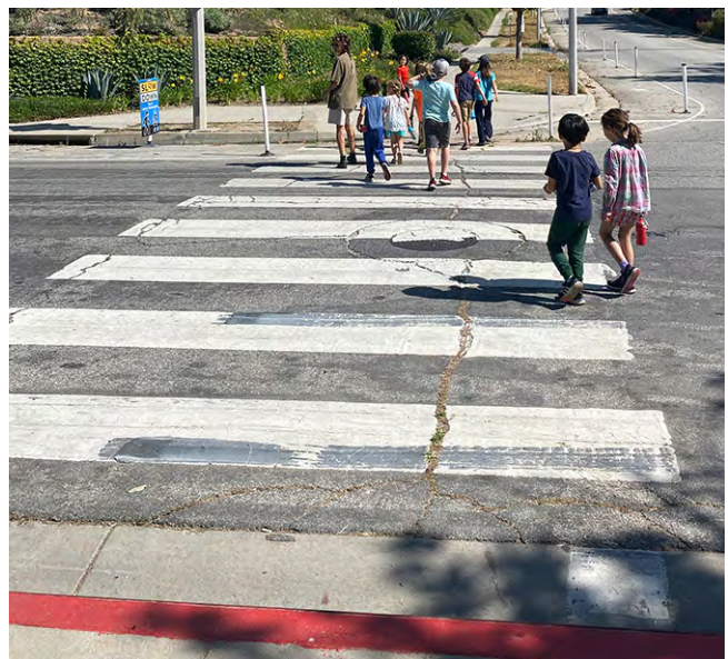
No curb ramp at the continental crosswalk on Loma Alta Drive and Sunset Ridge Road.
