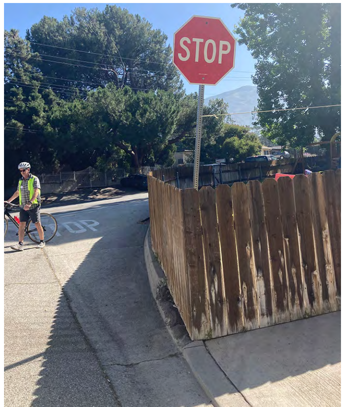
A stop sign behind the fence of a private residency blocks visibility.
