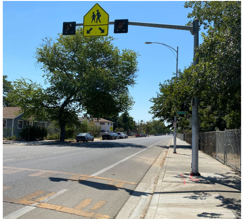
A School Zone HAWK pedestrian beacon on A Street/Calaveras Street at the marked yellow school zone crosswalk are one of the safety features along this route.
