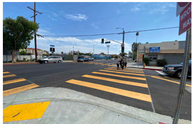
Pedestrian infrastructure treatments at the Main Street/West 76th Street Intersection
